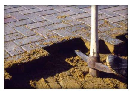
Figure 6. Prying out the remaining pavers
