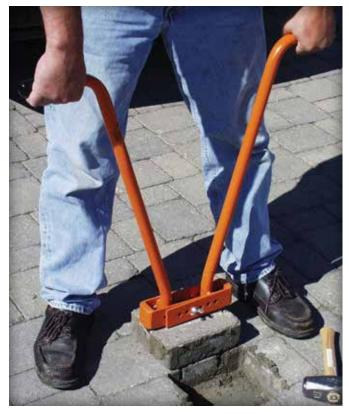
Figure 5. Using a paver extractor to remove a paver
