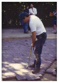
Figure 13. Adjusting joint spacing and alignment.
