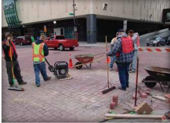
*Figure 15 and 16. Reinstated pavers leave no ugly patches nor do they weaken the pavement.*
