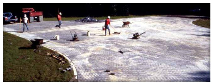
Figure 12. Excess sand swept from the finished surface will make the pavement ready for traffic.
