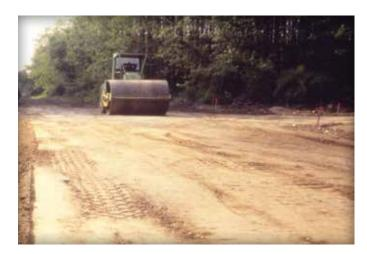
Figure 2. Compacting the soil subgrade.
