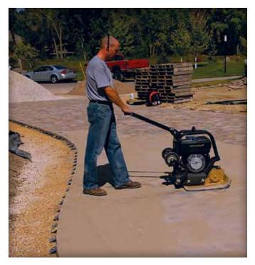
Figure 11. Vibrating sand into the joints.
