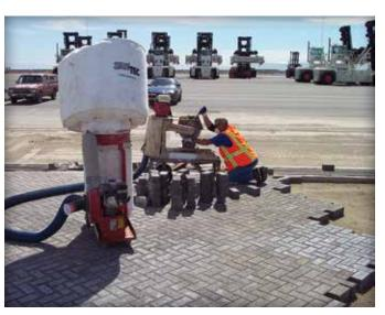
Figure 8. Saw cutting pavers.
