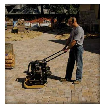
Figure 9. Compacting the pavers and bedding sand.
