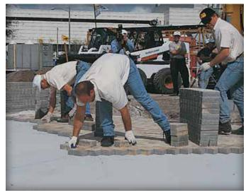
Figure 7. Placing the concrete pavers.
