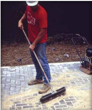
Figure 10. Spreading and sweeping joint sand.
