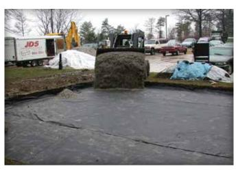
Figure 3. Application of the geotextile under aggregate base.
