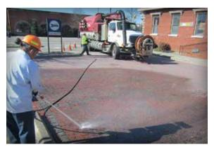
Figure 19. Power washing requires a little practice to minimize jointing stone removal.
