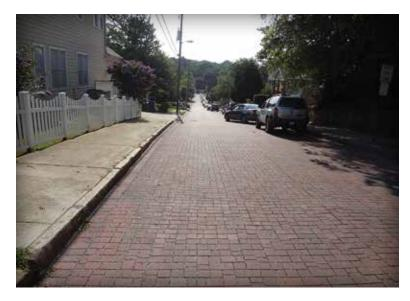
Figure 1. PICP is seeing increased use in municipal streets to reduce stormwater runoff, local flooding, storm pipe upsizing, and combined sewer overflows. These streets are in Atlanta, GA.
