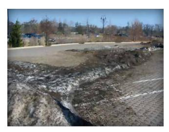
Figure 24. This is an example of snow that should have been deposited on a grassy area. If such areas are not available, then vacuum clean the PICP in the early spring.
