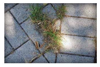
Figure 9. Weeds indicate sediment accumulation and lack of surface cleaning to remove it.
