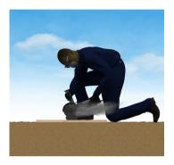
The best tool to cut pavers is a masonry saw but angle grinders are also commonly used in South Africa. Either way, good quality diamond blades are non-negotiable.
